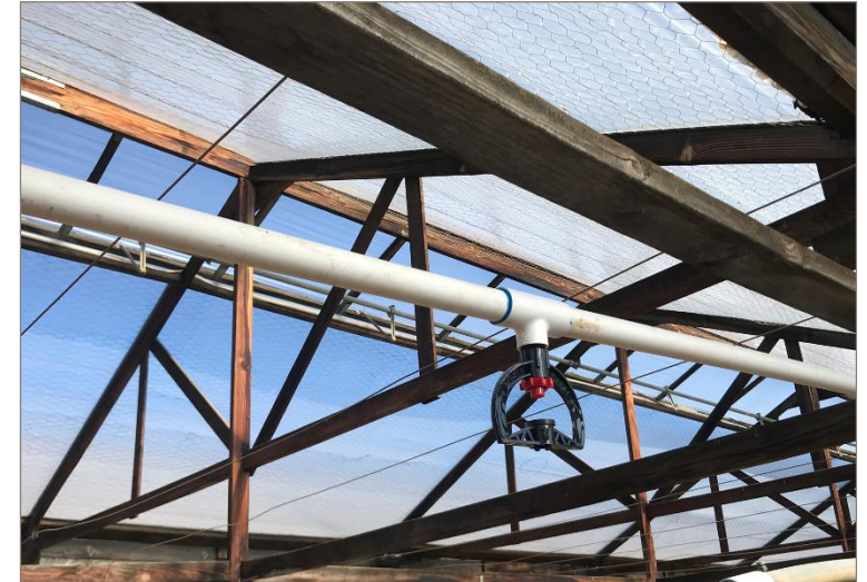
New sprinkler heads and pipes installed
