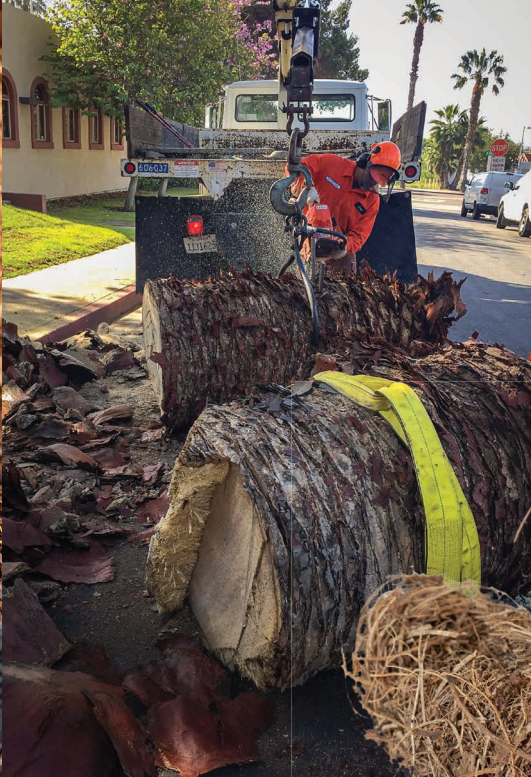
Tree removal due to infestation.
