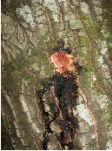
Figure 131. Bark of this coast live oak was chipped away at the point where wetwood ooze originated to show a small area of water-soaked, necrotic bark. Foul-smelling, clear liquid streamed from the area for several seconds when the bark was cut open.
