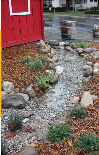
Figure 4. This newly planted garden makes it easy to see the downspout from the roof directing water to the garden. Stones are used to stabilize the area where water enters the garden and to prevent erosion. Source: M. Myers
