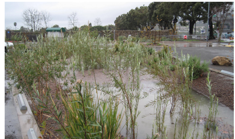
Figure 7. Runoff from surrounding areas flows into the rain garden basin, inundating the plants in this public landscape and parking area. Source: M. Myers
