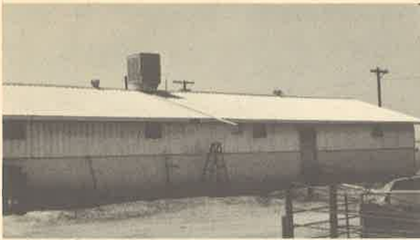
A well-insulated central farrowing house provides year-round comfort. Note extremely flexible ventilation (windows, two-speed fan on cooler with water optional, and ridge top ventilators) — very workable house for all seasons.
