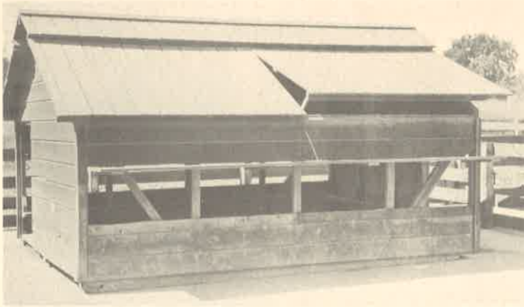
This small type hog house will take care of two sows and their litters. It is portable and provides good protection from sun and rain.
