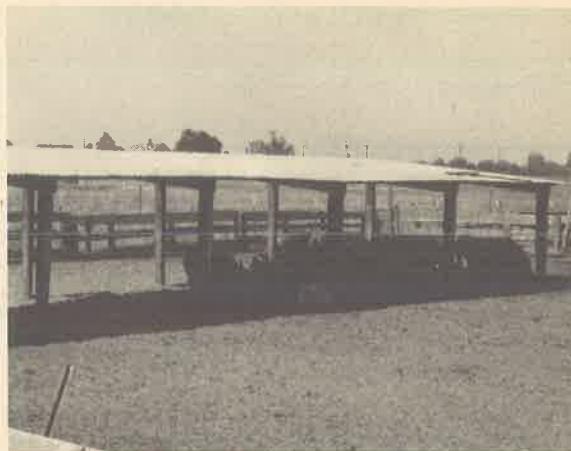
This dirt lot, located in an area of low rainfall and on sandy soil, functions well as a finishing facility. Sprinklers settle dust and cool the area in summer.
