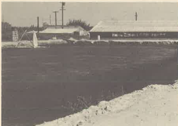
This is the first of three storage ponds used to process liquid waste.
