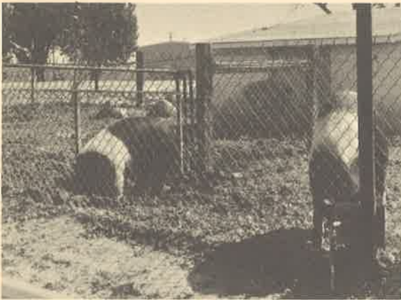
A diamond mesh fence.
