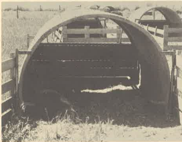
An open-front unit is limited in use to spring and fall farrowings. Construction is of corrugated metal. Straw is used for bedding, and guard rails protect pigs from overlay. This house is 6 feet wide, 5 feet high, and 8 feet long.
