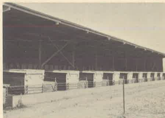
From 300 to 500 pigs can be grown out in this open-fronted fattening barn. Higher labor and water requirements for cleaning these solid floor pens will limit interest in this type of building. Note large capacity self-feeders. One feeder space for 4 to 5 pigs and one waterer per 30 head will adequately meet feed and water space requirements.
