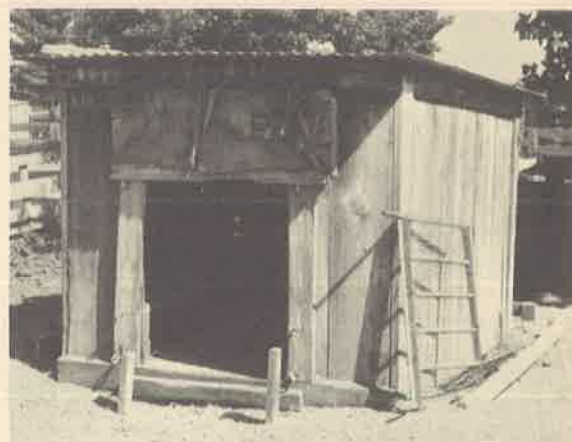
This individual farrowing house can be used seasonally or, in milder climates, year-round. The panel is used to lock the sow in when desired, and a burlap flap is used to reduce drafts. Interior features include guard rails, a heat lamp, and wood floor. This house is 6 feet high, 6 feet wide and 9 feet long.
