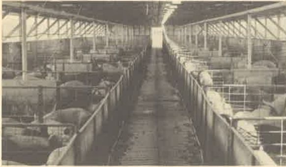
This slatted floor building features adjustable plastic side curtains and concrete slats.
