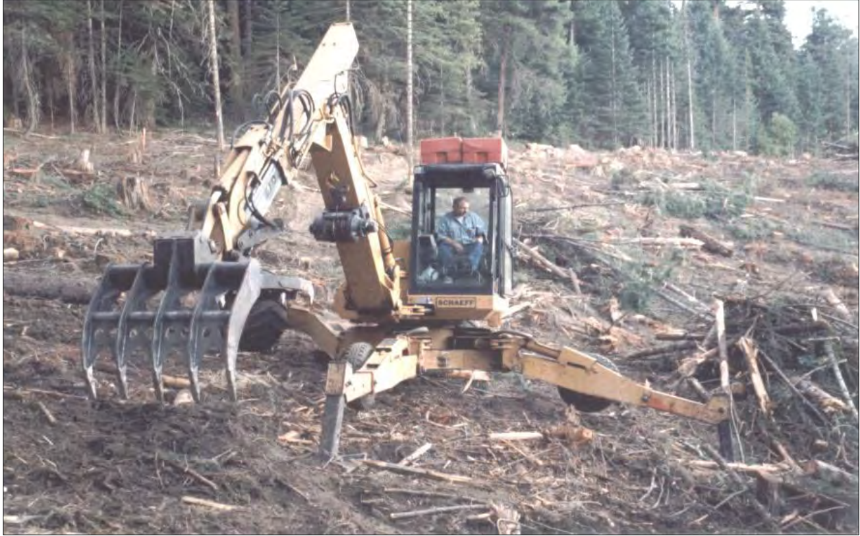
Figure 7.9 Spyder site preparation machine.
