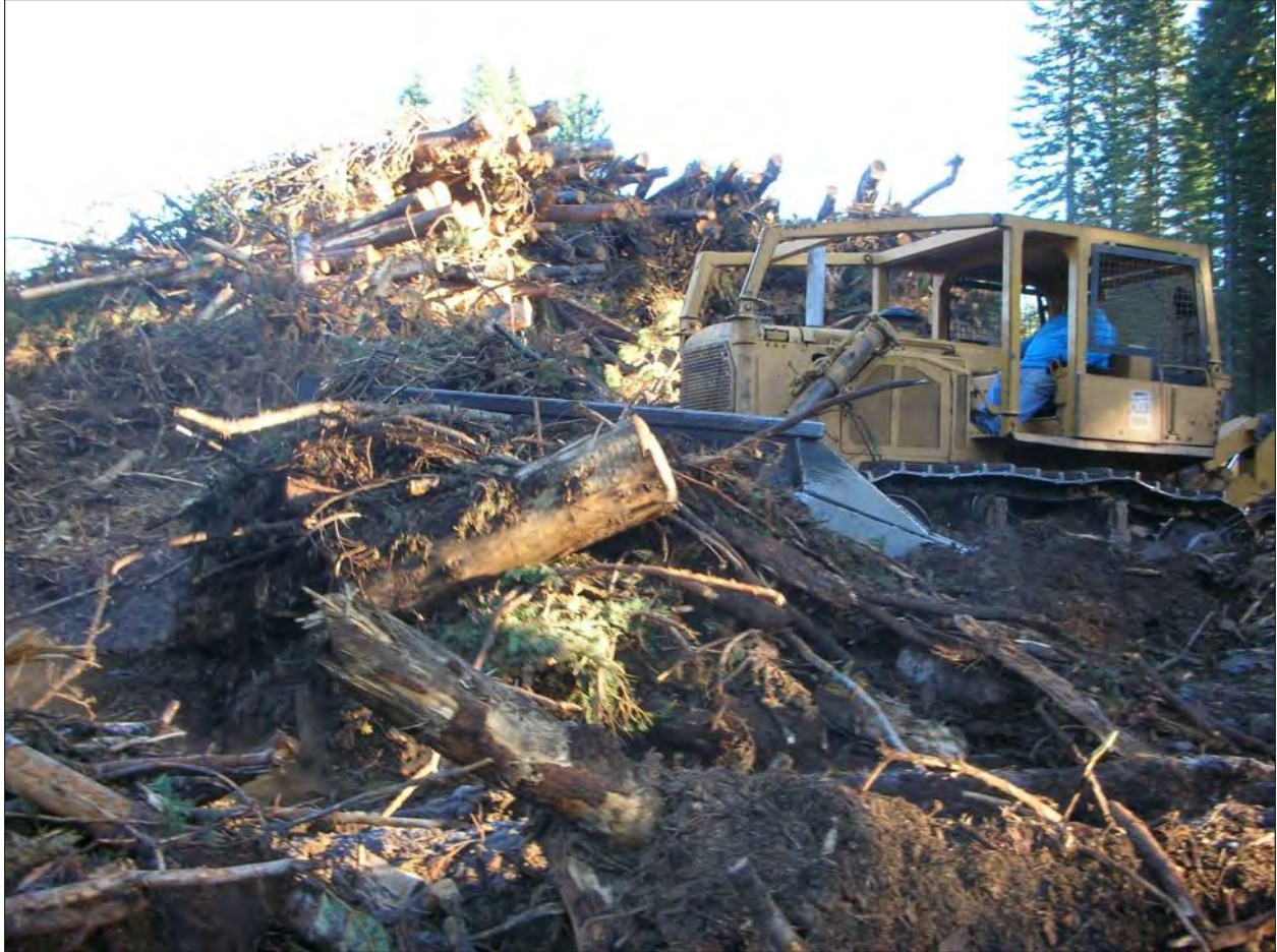
Figure 7.7 V-Blade clearing landing slash for planting.
