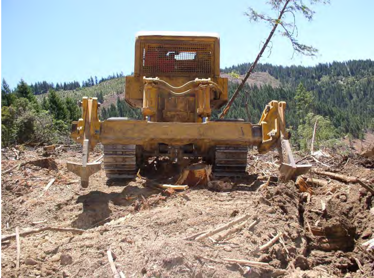
Figure 7.4 D8 with Winged Sub-soiler shanks.
