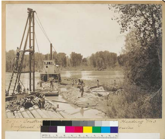
A CREW ERECTING A DIKE VICINITY THIRD HEADING OF FLOODED IMPERIAL CANAL, CIRCA 1905 PHOTO-JOSEPH LIPPINCOTT SOURCE ONLINE ARCHIVE OF CALIFORNIA
