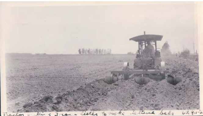
Three photos showing lettuce farming techniques from 1925. 1: "Floating" or leveling the field 2: Using a "Lister" to make lettuce beds 3: Bed shaper and seed drill for planting lettuce. There was a proliferation of "homemade" planters in the pictorial archives but this one seemed most representative. Courtesy ICCE Collection: Cecilia Olea, Annette Tietz.
