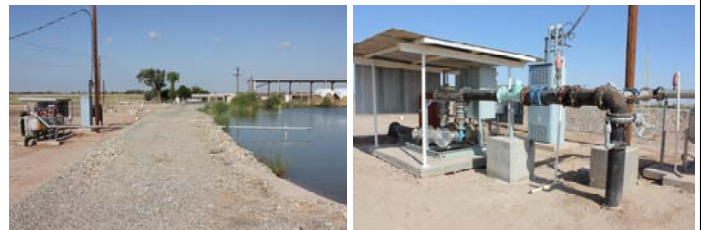
Photos above: Reservoir water can be filtered and pumped underground to any research plot on the DREC. Gravity irrigation system also utilizes underground piping. Photos courtesy AI Robertson.
