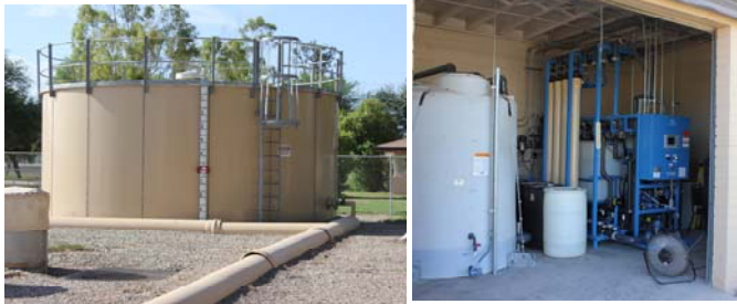
2012 photos of Domestic water plant renovation. Al Robertson
