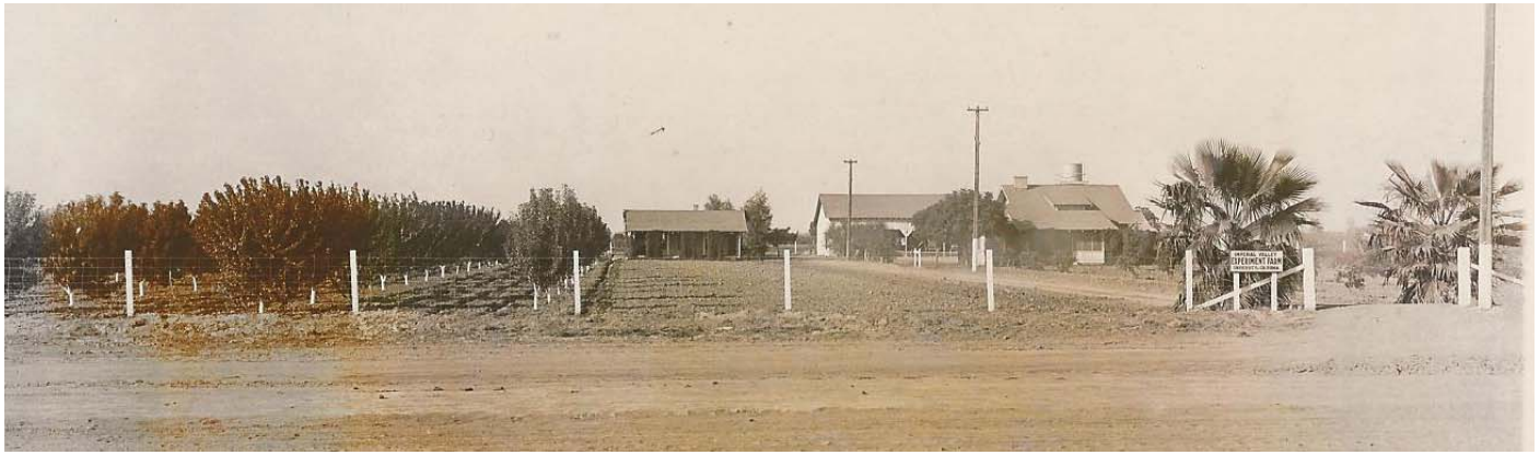
The 1915 photo above is the earliest picture found in the archives at the UC DREC. At the end of the entrance driveway, four were structures were built: Main residence, hired hand residence, office building and a barn. Notice the water behind main residence. Entrance sign reads:
