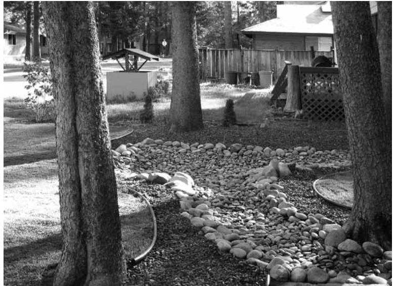
This above-ground infiltration system captures, stores, and infiltrates roof runoff.
