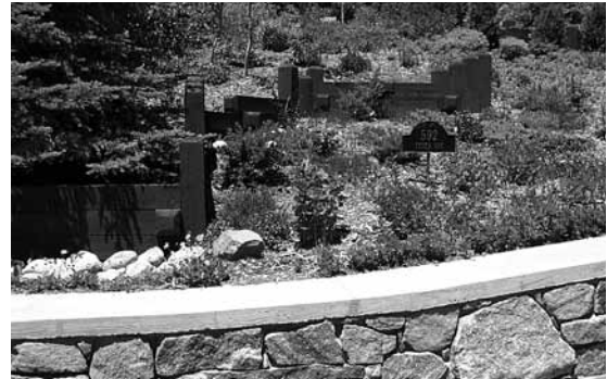
Below, a rock-faced retaining wall with nearly level planting terraces above it
