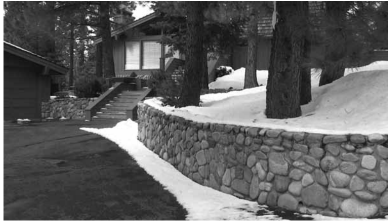
Above, a rock-faced retaining wall adjacent to a driveway.
