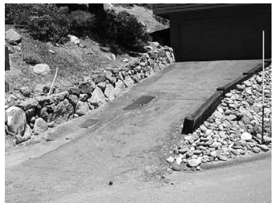
At left, the pervious pavement is laid on top of a permeable subgrade of gravel. The driveway below has a steep slope and very little space at the foot of the slope for an infiltration system.
