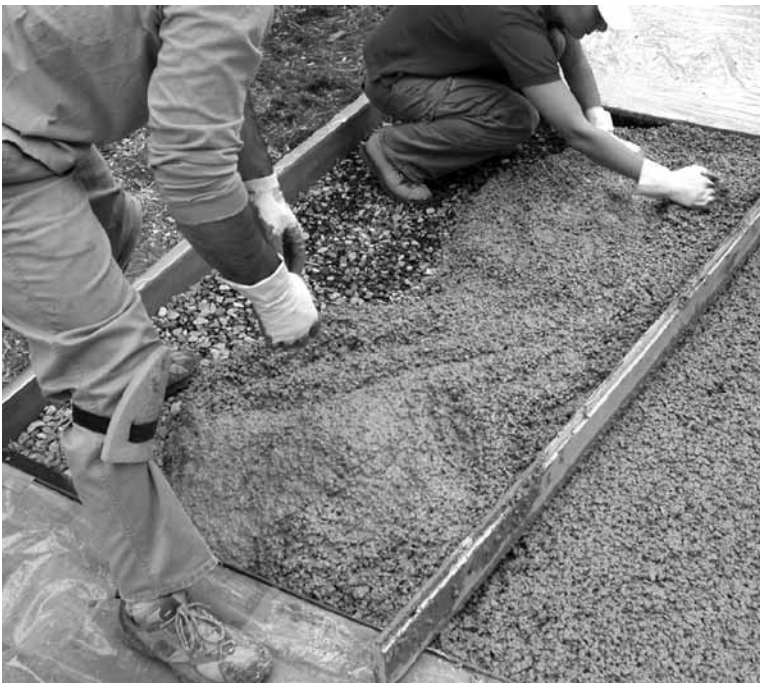
At left, the pervious pavement is laid on top of a permeable subgrade of gravel. The driveway below has a steep slope and very little space at the foot of the slope for an infiltration system.
