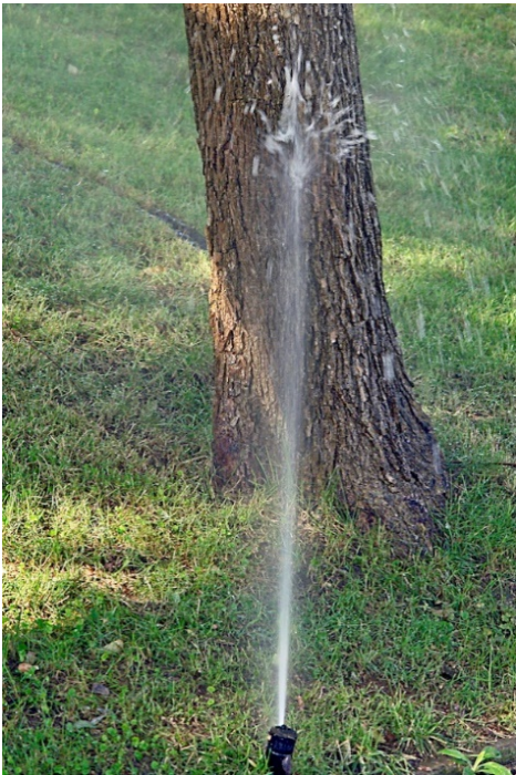
Sprinkler hitting trunk
