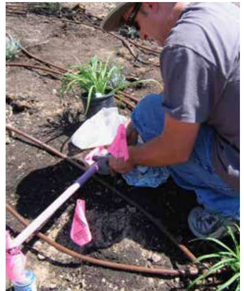
The brown tubing has drip emitters built in. Photo by Elaine Applebaum
