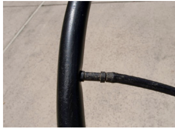
1/4-inch tubing inserted into 1/2-inch tubing
