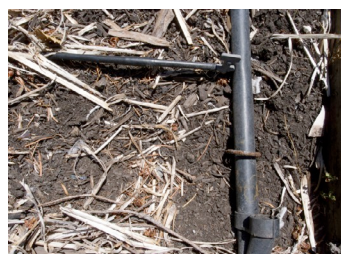
Staple securing the 1/2-inch tubing
