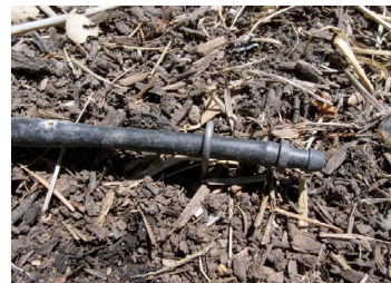
Staple securing the tubing
