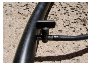
Valve inserted in 1/2-inch tubing
