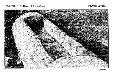
Fig. 1.—Salt log used on cattle range of Whitman National Porest. Smooth, twisted wire stapled every 4 inches is used, as shown, to protect the trough from gnawing by horses and porcupines.
