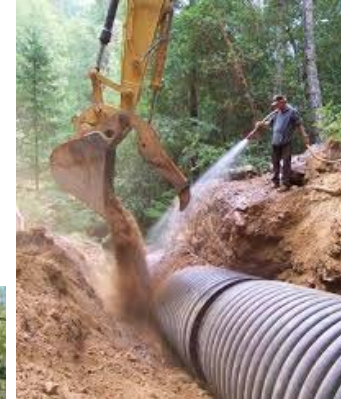
Water crossing upgrades
