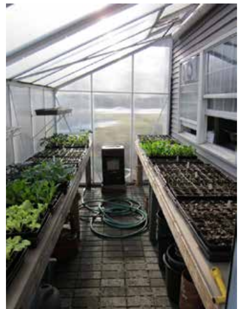
A lean-to greenhouse is easily accessible and allows for heat exchange between the house and greenhouse
