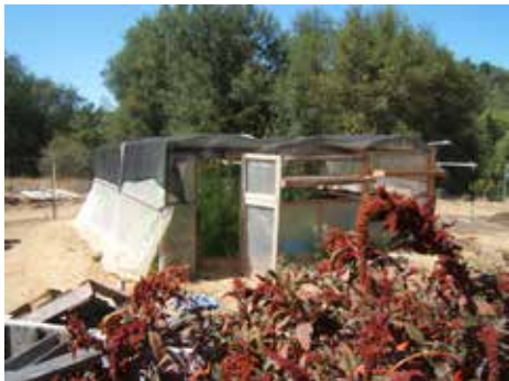
Shade cloth and large windows help cool a simple plastic covered greenhouse
