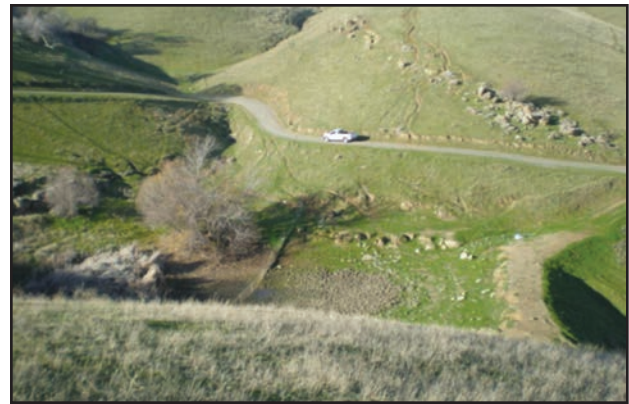
Pond D5 view 1, Contra Costa County, 2009 (pond dry; dam to right, fence in center; by P. Van Hoorn).
