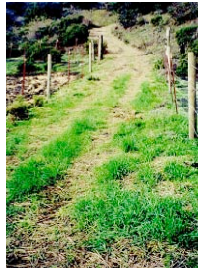
Roads not used in the winter can be “put to bed” for the season. This road has been seeded and will not be used again until the spring. Roads should be properly graded, seeded and mulched, to help prevent erosion. Seeding should occur before October 15 to ensure adequate growth before the winter rains.
