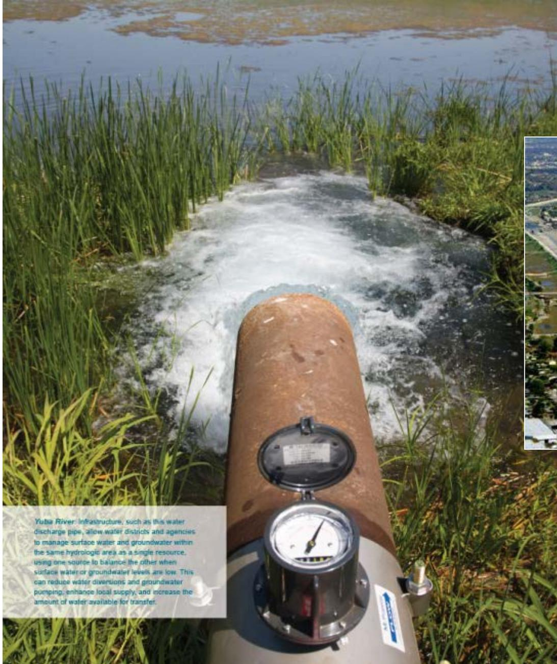
Yuba River infrastructure, such as this water discharge pipe, allow water districts and agencies to manage surface water and groundwater within the same hydrologic area as a single resource, using one source to balance the other when surface water or groundwater levels are low. This can reduce water diversions and groundwater pumping, enhance local supply, and increase the amount of water available for transfer.
