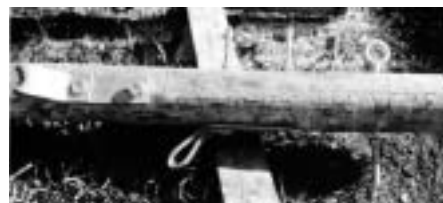
guy line anchor used on ginseng trellising (left & centre of picture): strong, but expensive. Right: forged steel loop used to anchor cross cables.
