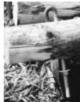
This is an edge pole, with guy line wrapped around the top and fastened with two cable clamps, as is the cable running across the field. The cable parallel to the line of poles is run through the gap between the guy line loop and the pole. Cables between the poles are simply looped around the parallel cable and clamped.
