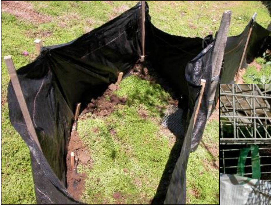
Corral Trap using Silt Fence
