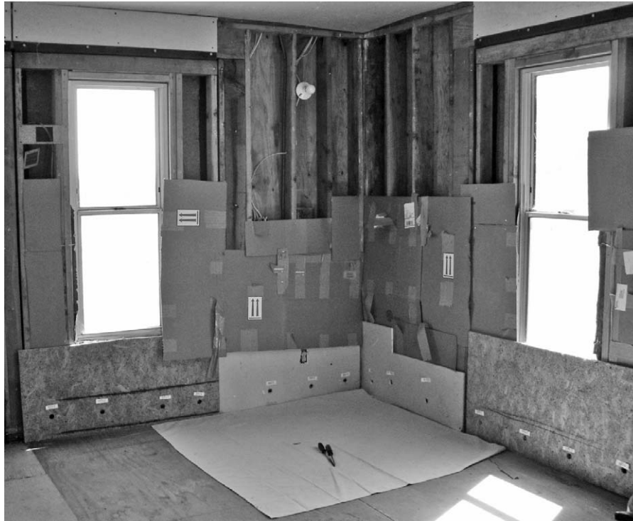
Figure 3.—View of bore holes used for borescope insertion into experimental wall voids used for the simulated field assessment of identification accuracy. Each void was designated either as an internal void or an external void containing insulation materials and held one of seven sample types within.
