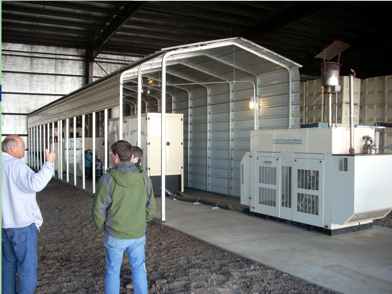
Community Power Corp BioMax 50 kWh CHP at Dixon Ridge Walnut Farm, Winters, CA
