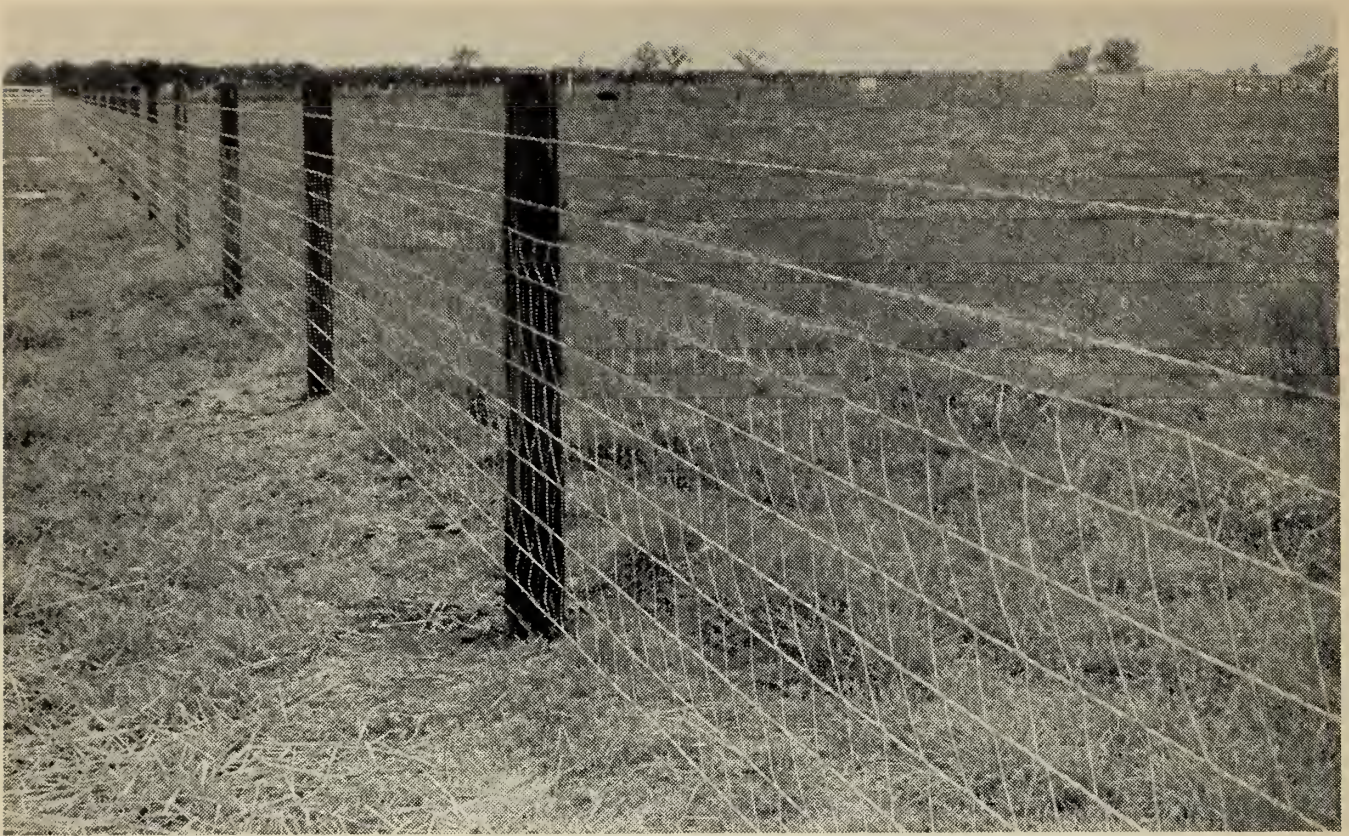
“Sheep-tight” fences such as that shown above should be made of woven wire, with barbed wire above to protect the woven wire.
