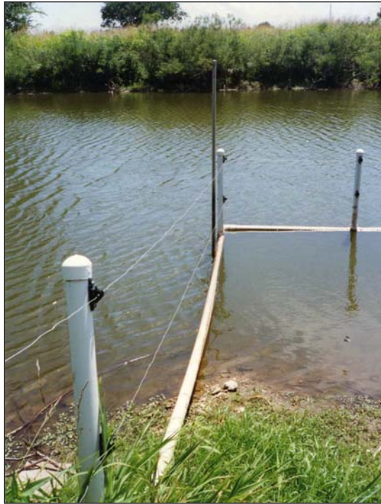
Floating pipe and electric fencing limit livestock access to the pond. By A. E. Beetz, 2005.
