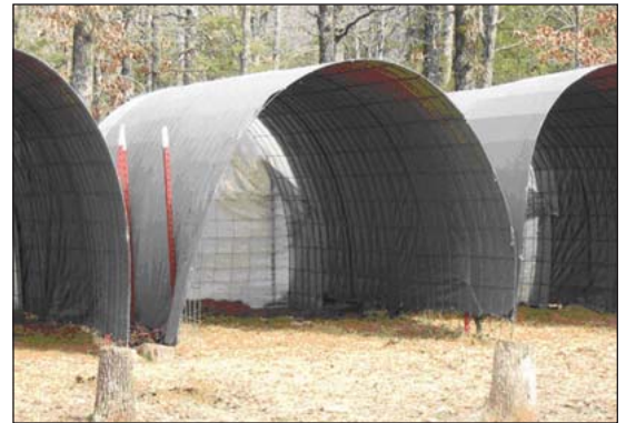
Cattle panels with a tarp stretched over them provide adequate shelter for goats.
