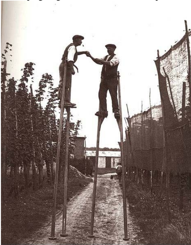
Working the hops trellises in the 'olden' days
