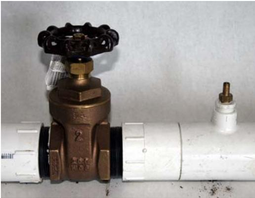
Figure 1. A gate valve with a Schrader valve allows pressure to be adjusted and monitored in an irrigation block, but the valve must be adjusted manually to compensate for changes in upstream pressure.
