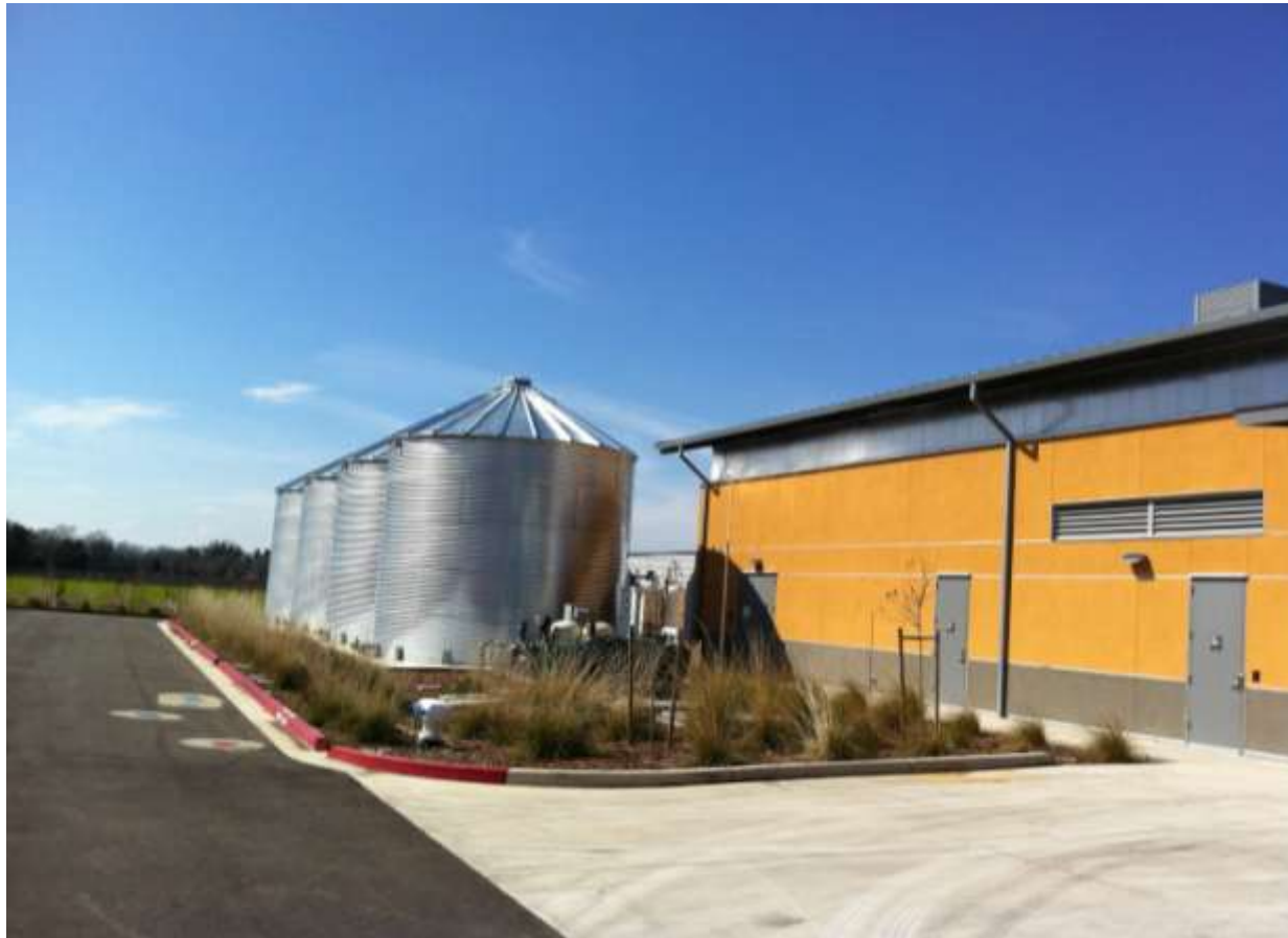
Rain water harvest, bio-swale treatment, storage and treatment system at UC Davis
