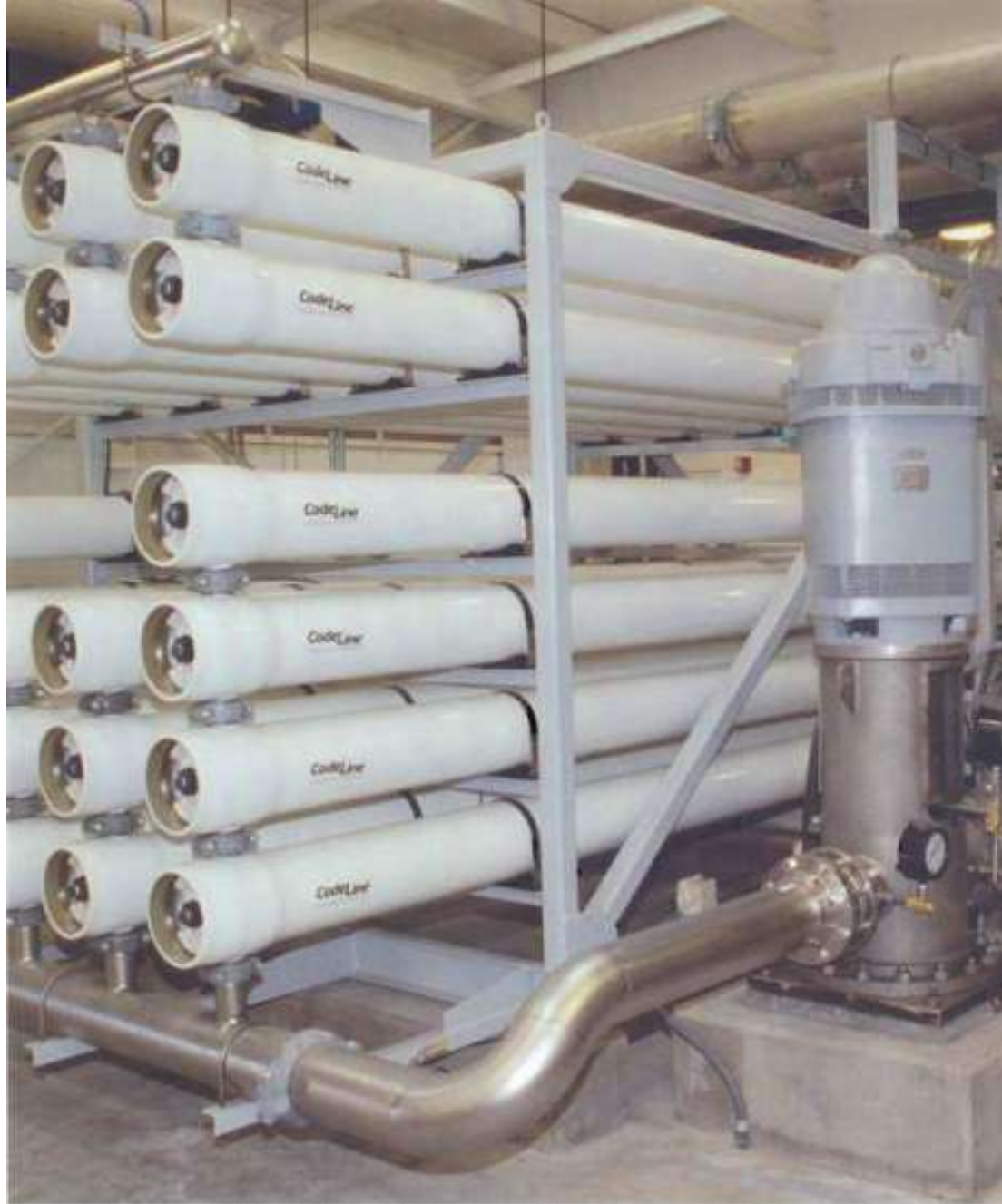
Swooswater Authority customers benefit from this desalination facility that treats brackish or saline groundwater. About 24 groundwater desalting plants operate in California and provide water for municipal purposes. The total capacity of these plants is approximately 79,000 acre-feet per year. (DWR photo)
