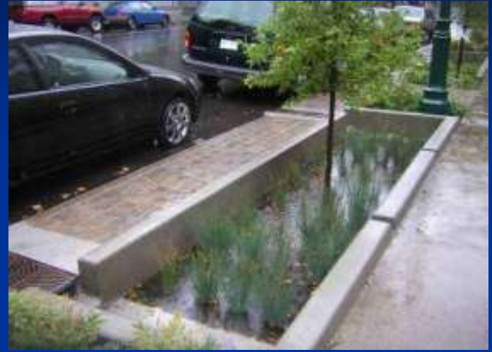
SW 12 th Avenue Green Street
