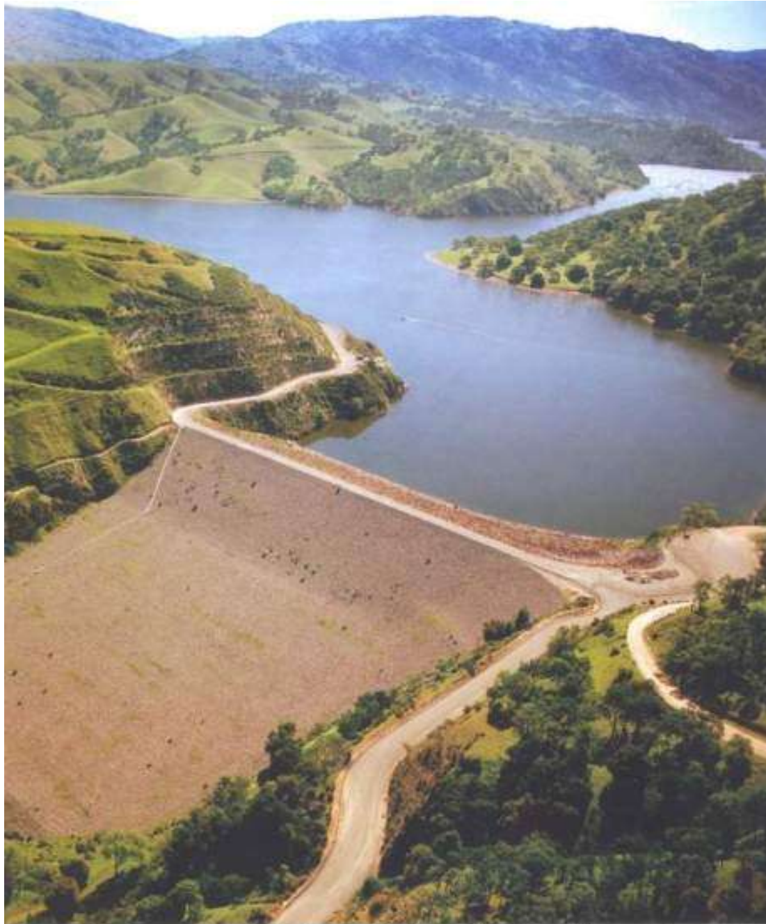
Surface storage plays an important role in California where the pattern and timing of water use does not always match the natural runoff pattern. Contra Costa Water District pumps high quality water into its Los Vaqueros Reservoir and uses it to lower salt content of water it pumps from the Delta. (DWR photo)
