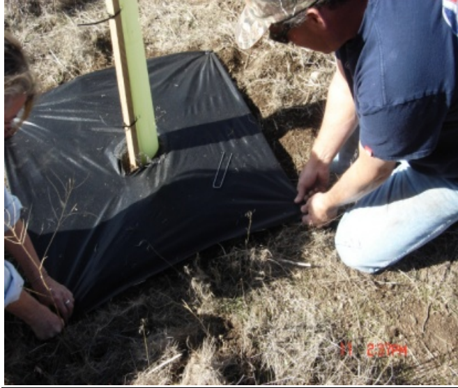
Securing Corners of Tree Mat with Staples
