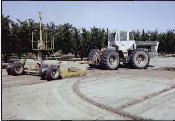
Fig. 5.2. Laser leveling a field in preparation for planting.
