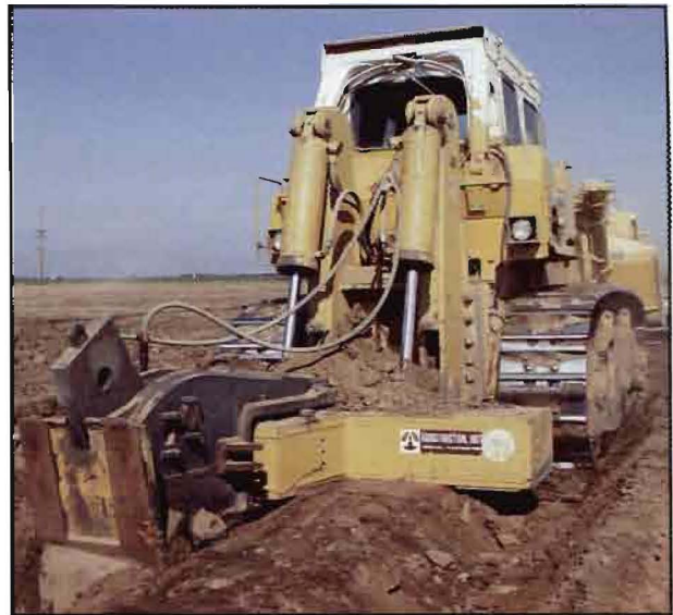
Fig. 5.1. Deep ripping an orchard site to break up a hardpan layer.
