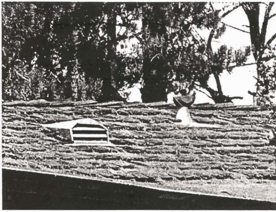
Figure 7. ~ An example of a dormer-type through roof vent that would be vulnerable to both wind-driven rain and flames and embers from a wildfire. Debris from nearby pine trees and the untreated shake roof also pose significant problems for this structure.
