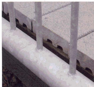
A composite deck board with channeled configuration was used in this 'open framed' deck.
