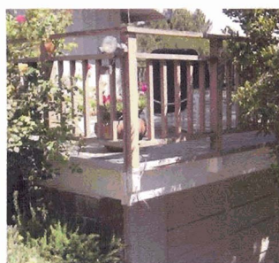
In an enclosed deck the supporting framework does not show.
