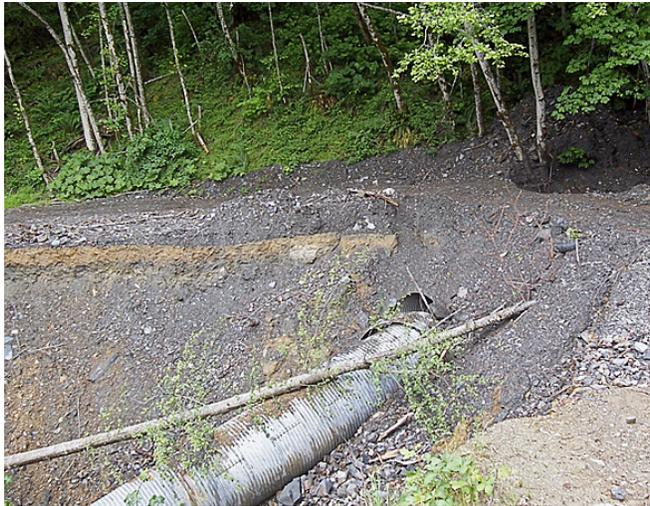
**Figure 1.** Culverted stream crossings may plug during storms. Diverted stream flow then crosses the road and erodes the fill slope.
