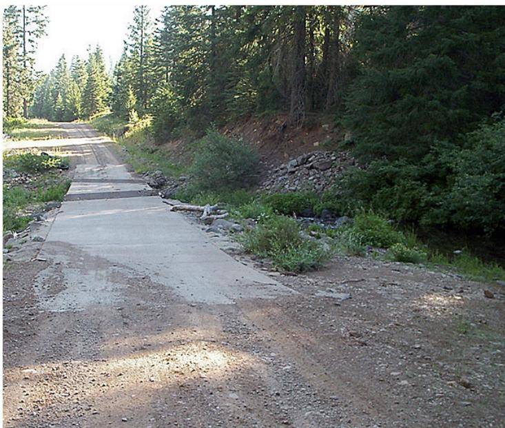
**Figure 14.** Concrete ford on bedrock outcrop in perennial stream.
