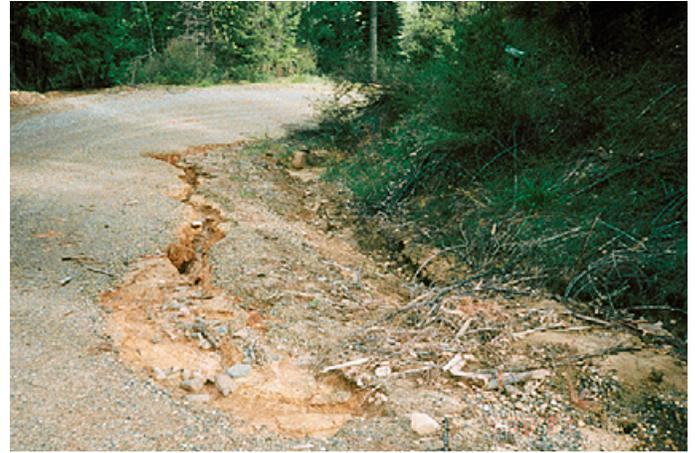
**Figure 9.** This ditch and road surface erosion was caused by inadequate spacing of ditch relief culverts. *Photo:* Susie Kocher.
