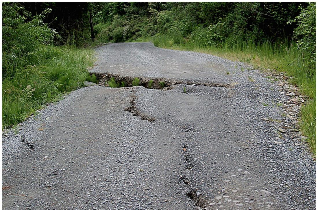
**Figure 21.** Cracks appearing in the road surface, especially at the edges of fills, are a sure sign of an impending failure or landslide. The horsetail growing in these cracks indicates that the source of the problem is groundwater seeping through the road bed. *Photo:* Richard Harris.
