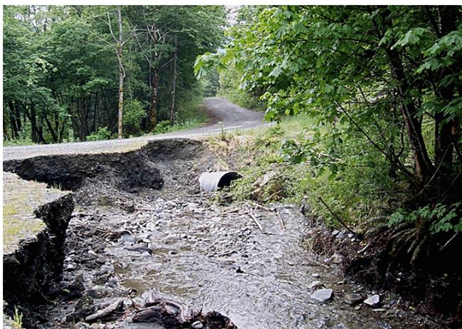
**Figure 18.** This culvert plugged with debris during a storm. Although it is still in place, the swirling water and debris caused extensive erosion of the road and the adjacent old log landing. This type of failure is common on older “legacy” roads where crossings were not adequately designed to pass 100-year flows plus debris and sediment. In many cases, the culvert will be displaced and transported downstream.
