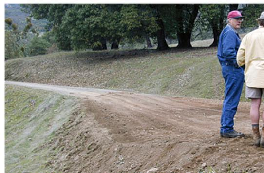
**Figure 11.** This rolling dip has a gentle increase in grade going left to right and a reverse grade (where people are standing) to direct water off the road at the dip. *Photo:* Gary Nakamura.
