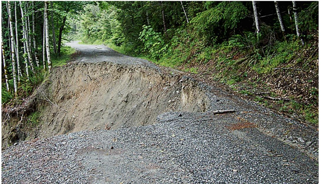
**Figure 3.** Stream undercutting at the base of the slope below the road caused this landslide.
