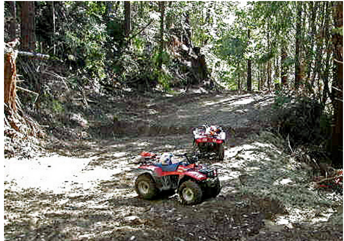
Figure 9. Water bars installed on a road after timber harvesting. Source: Angela Wilson, Central Valley Regional Water Quality Control Board.
