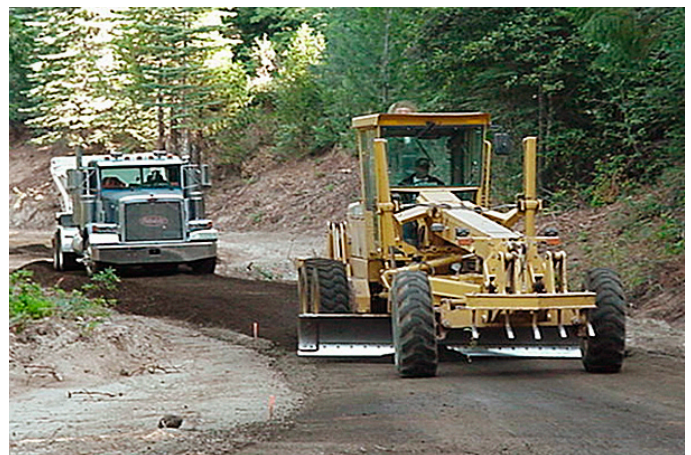
Figure 33. A grader spreading the gravel on the road surface placed by a dump truck. Source: Joe Hoffman, Plumas National Forest.
