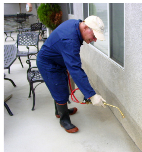
Figure 1. Applying a fan spray 1 foot up and 1 foot out from a house foundation.
