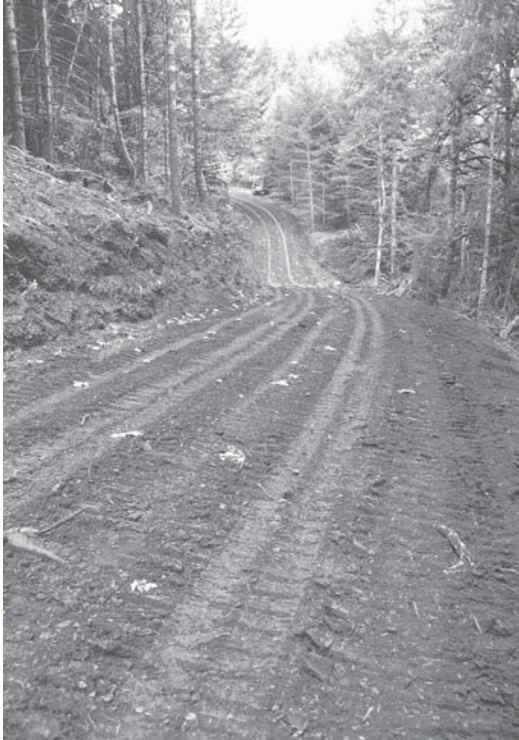
Figure 4-12. Native-soil-surfaced road.
