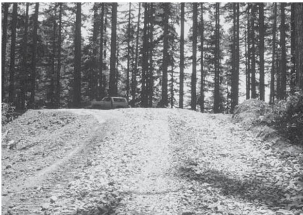
Figure 4-13. Rock-surfaced road.
