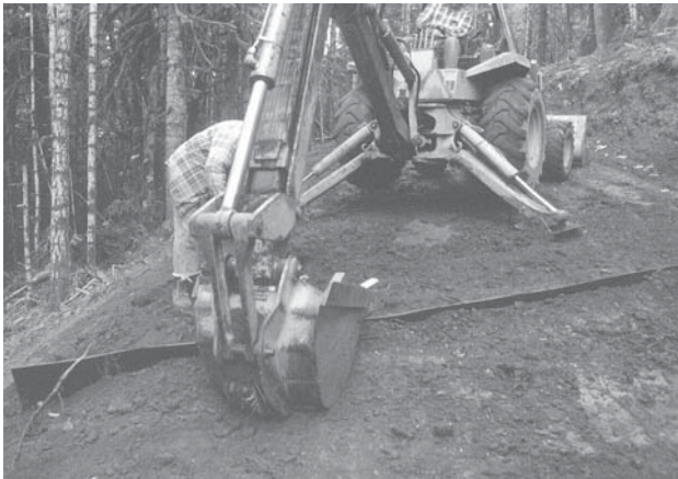
Figure 3-11. Installing a rubber water bar
