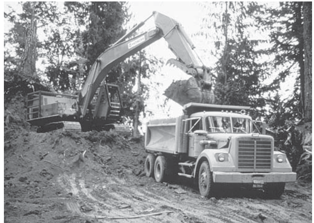
Figure 4-7. Hydraulic excavator excavating roadway material.
