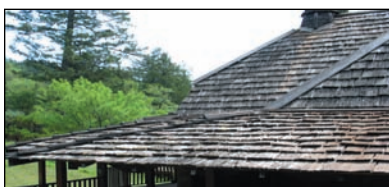
Wood shake roofs are prime receivers of burning embers -- and prime reasons that houses burn down in wildfires.
