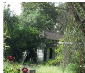
This home is completely surrounded by flammable vegetation, making it impossible for firefighters to defend it.
