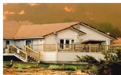
Enclosing the underside of your deck will keep burning embers out.
