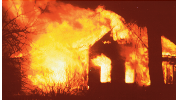
DIRECT FLAME CONTACT caused this building to be lost.
