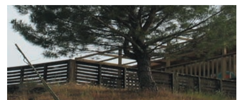
A wood fence can carry a fire right to your deck and house. Separate a wood fence from your house by a metal gate or an open space.
